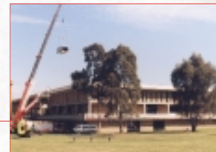
Installing the Chiller
