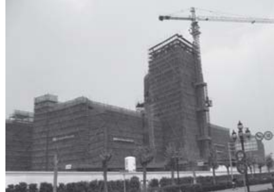
Shanghai Jiao Tong University Library under construction
